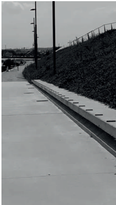
Figure 4.3: Pig's ears are a common design element to deter unwanted skateboarding. The image shows a concrete block in the Jardin du Musée des Confluences, Lyon (France). Photo: Smaniotto, 2018.
