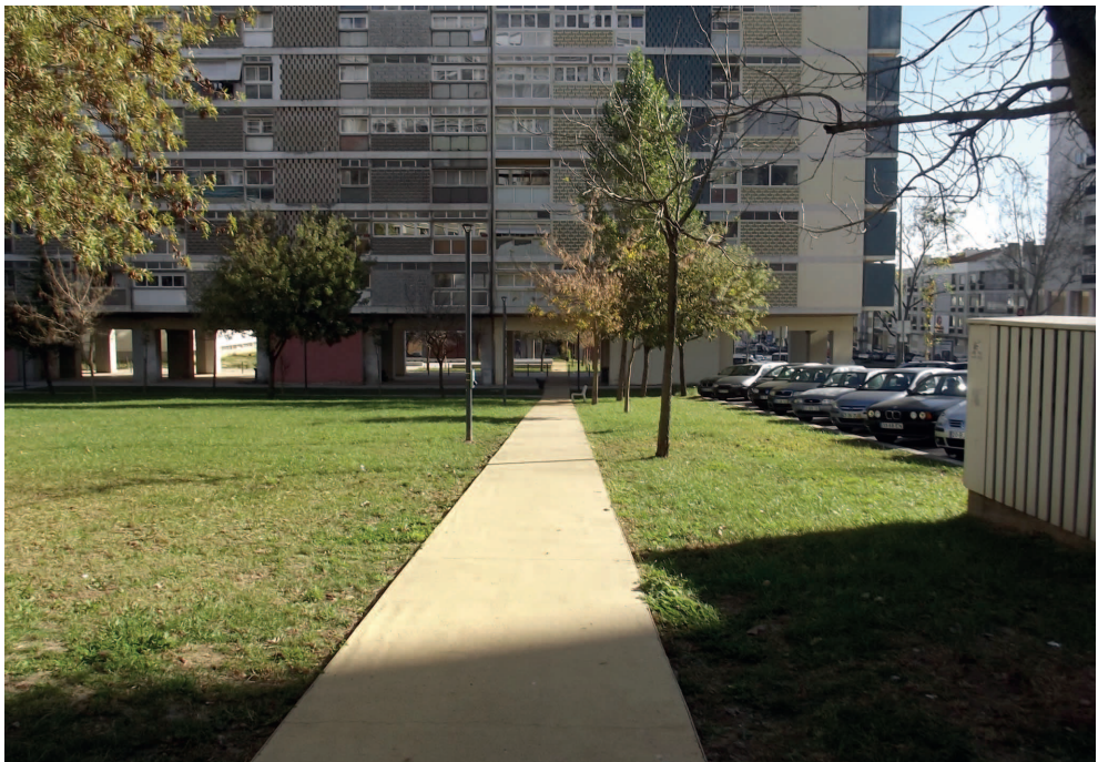
Figure 5.1: Typical high-rise building raised on pilotis; this design helps to create the sense of fluidity in Alvalade. Photo: C3Places Archive, 2020.
